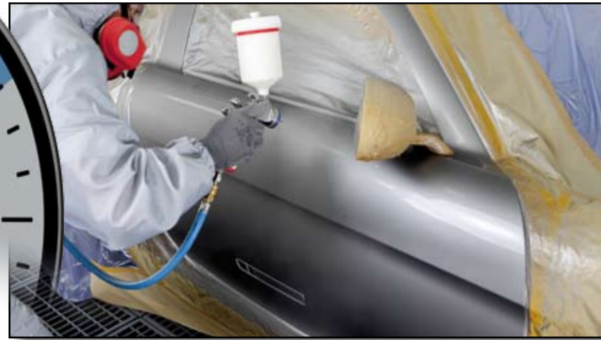
Applying the 2K Special Matt ready to use clearcoat mixture in two carefully controlled overlapping coats with inter-coat flash-off.
